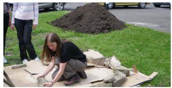
3 Build the spiral up in layers. Position stones to keep each layer relatively flat so the following layer is more stable.
