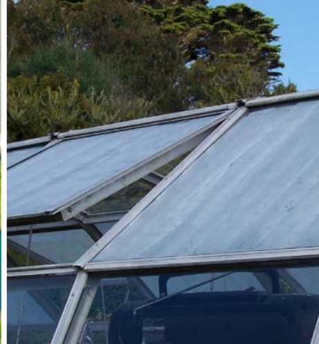
Use green mesh or 'shading wash' to keep temperature down in summer, but not reduce light too much.
